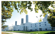
The Factory Building of the F-class Gas Turbine Large-capacity Flue Gas Waste Heat Deep Utilization Project
