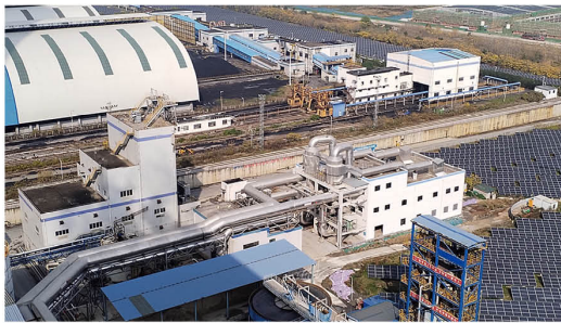
The Integrated Sludge Treatment Systems in Yueyang Power Plant
