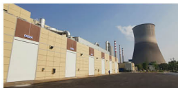
Luohuang Power Plant Sludge Disposal Center
