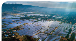
400 MW Photovoltaic Power Generation Project in Ruicheng County
