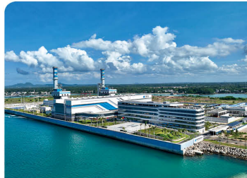
Yangtu Thermal Power Plant
