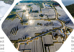
Shilin Solar Power Demonstration Area
