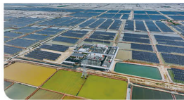
Shanyan 150 MW Photovoltaic Power Generation Project
