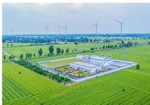
Puyang Wind Farm
