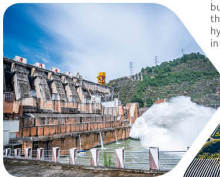
Manwan Hydropower Station
