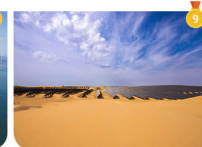
North United Power Co., Ltd. PV Power in the Desert (by Liu Haijun)
