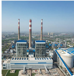
Shidongkou 1 st Power Plant
