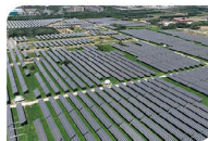
Qewo 300 MW Photovoltaic Project
